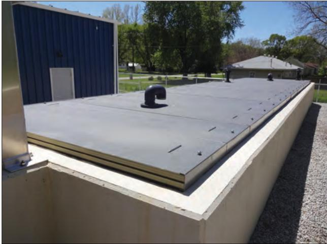
This photo shows the new covered sedimentation basin with hopper-bottom. Water is then pumped from the far end of this basin to the pressure filters.
