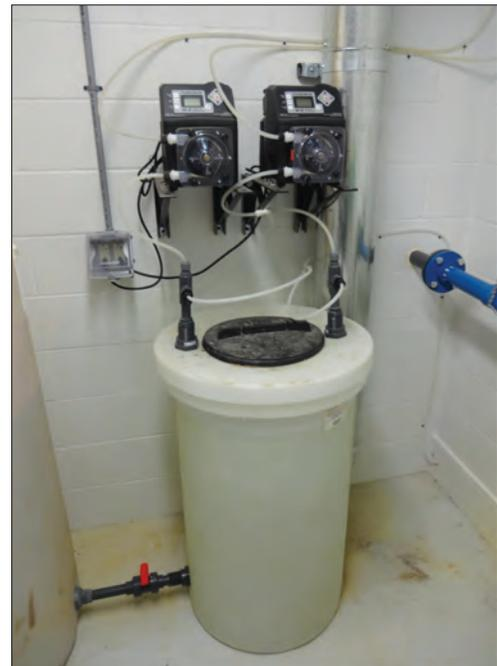
ProSeries-M peristaltic pumps are used for both pre and post-chlorination.
