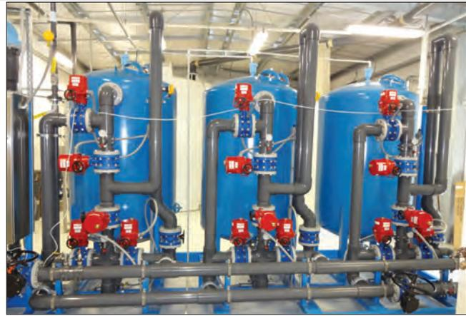
This photo shows the three Wigen pressure filters. This is the final treatment stage for removing any remaining iron and manganese from the water.
