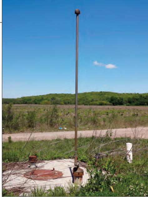
**This photo shows Well No. 3 with extended well vent. KDHE requires the elevation of the well vent be not less than two feet above the 100-year flood level.**
