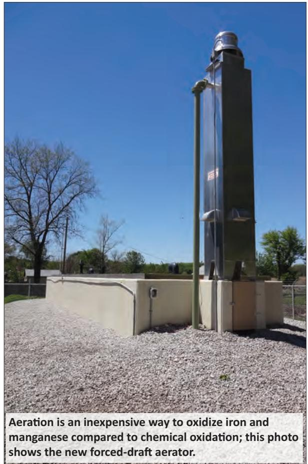
Aeration is an inexpensive way to oxidize iron and manganese compared to chemical oxidation; this photo shows the new forced-draft aerator.
